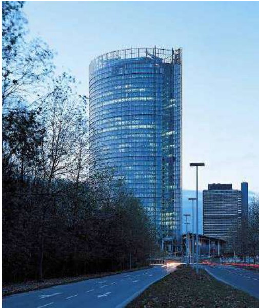
Figure 9.1 Post Tower in Bonn, by Murphy/Jahn, Inc. Architects. [Photo: Scheldebouw-Permasteelisa]
