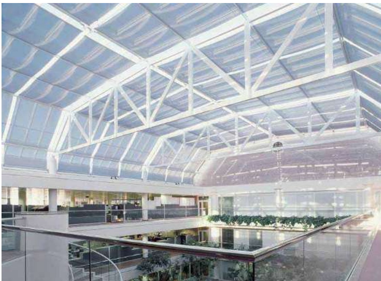
Figure 8.2 A bank building in Belgium, after the installation of blinds to cut the glare. [Photo: Hunter Douglas, Helioscreen]
