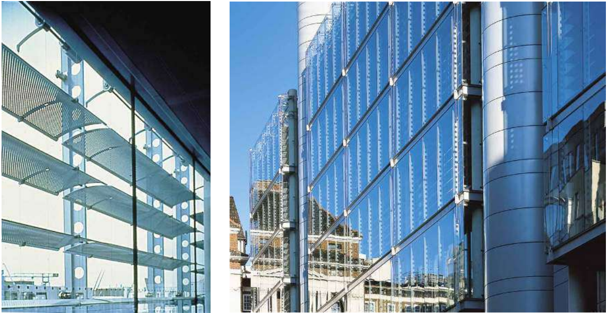
Figure 9.2 Solar shading blinds in the cavity of a double skin façade of The Helicon in London (Arch. Sheppard Robson). [Photo: Scheldebouw-Permasteelisa]
